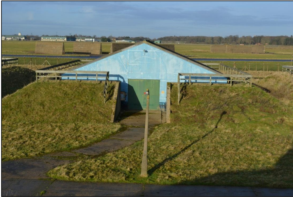
Figure 27: Outside of a ready-for-use store, originally used for Firestreak, former RAF Coltishall (note the blast walls to the rear of the store) (R Maguire 2012)
