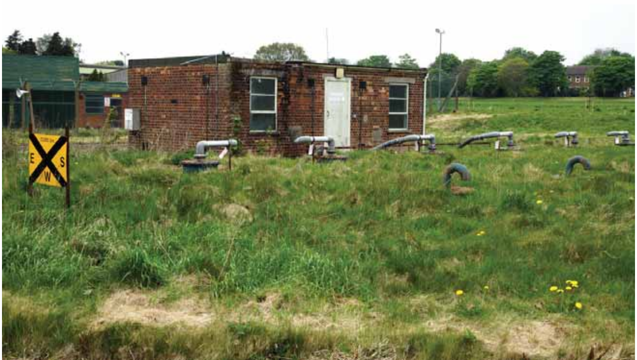
Plate 13: Aviation petrol installation (8), showing the positions of six buried tanks
