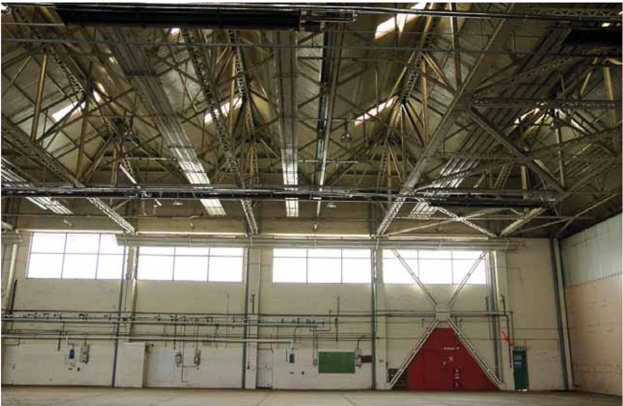
Plate 7: Hangar 1, internal side wall view showing the first full bay with wind bracing
