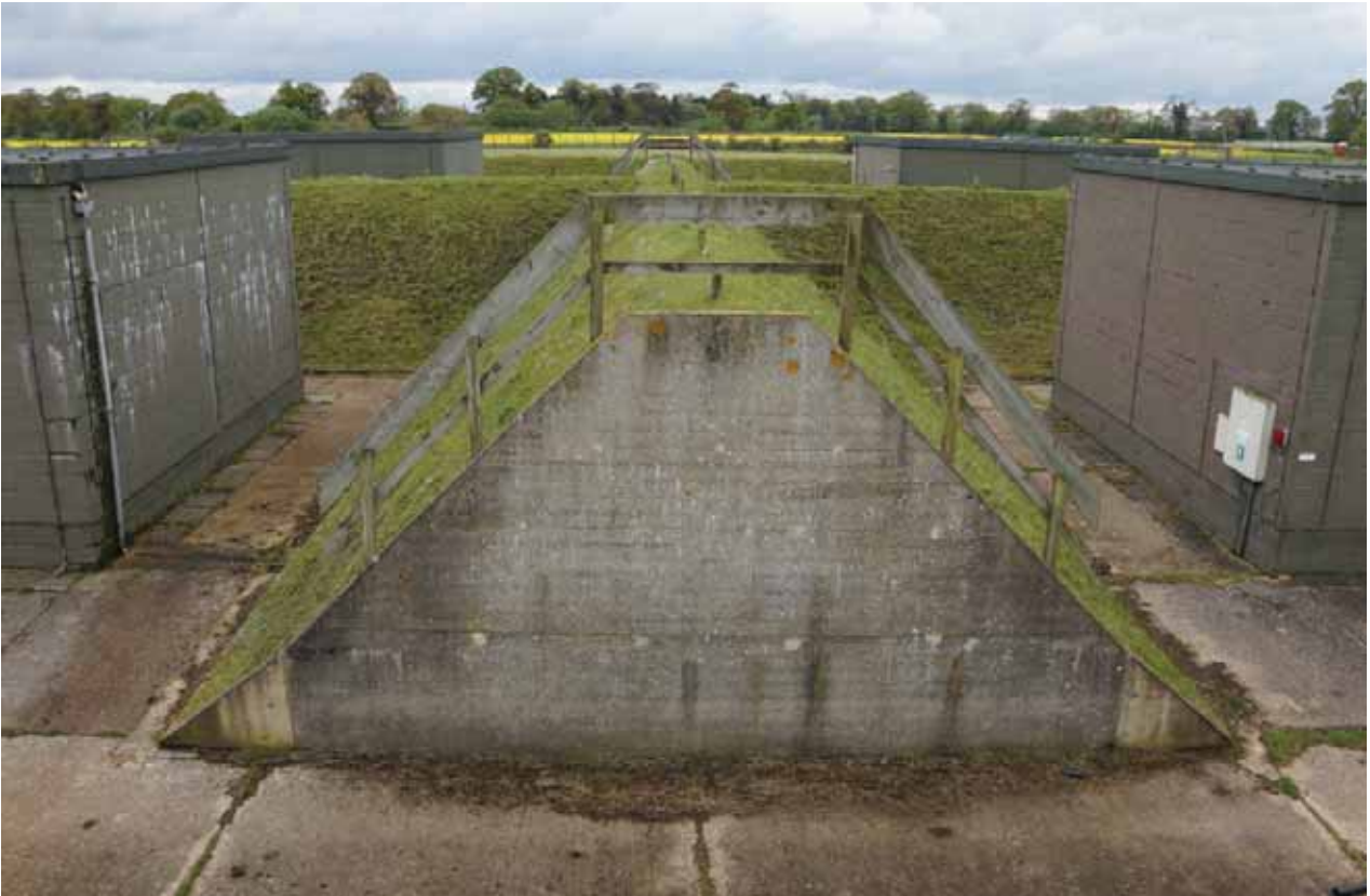
Plate 6: Bomb store, revetment detail separating a pair of storehouses (69)
