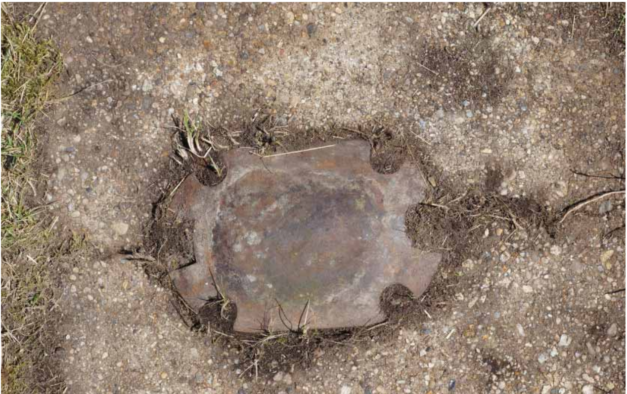
Plate 45: WWII 'Drem' C.5 flare path light fitting This is one of four similar fittings inside and outside the wire
