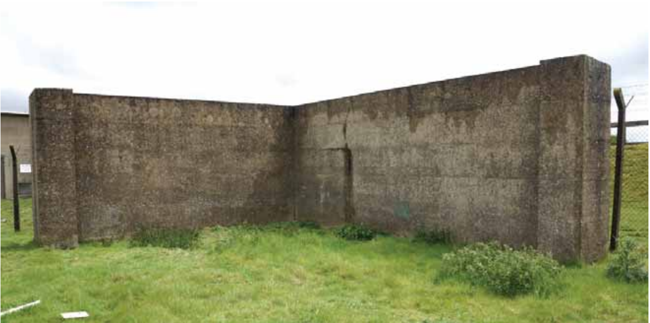
Plate 47: Monolithic concrete 'L'-shaped blast wall outside the wire It was built to protect an electrical sub-station (part of 256 sub-station 'K')
