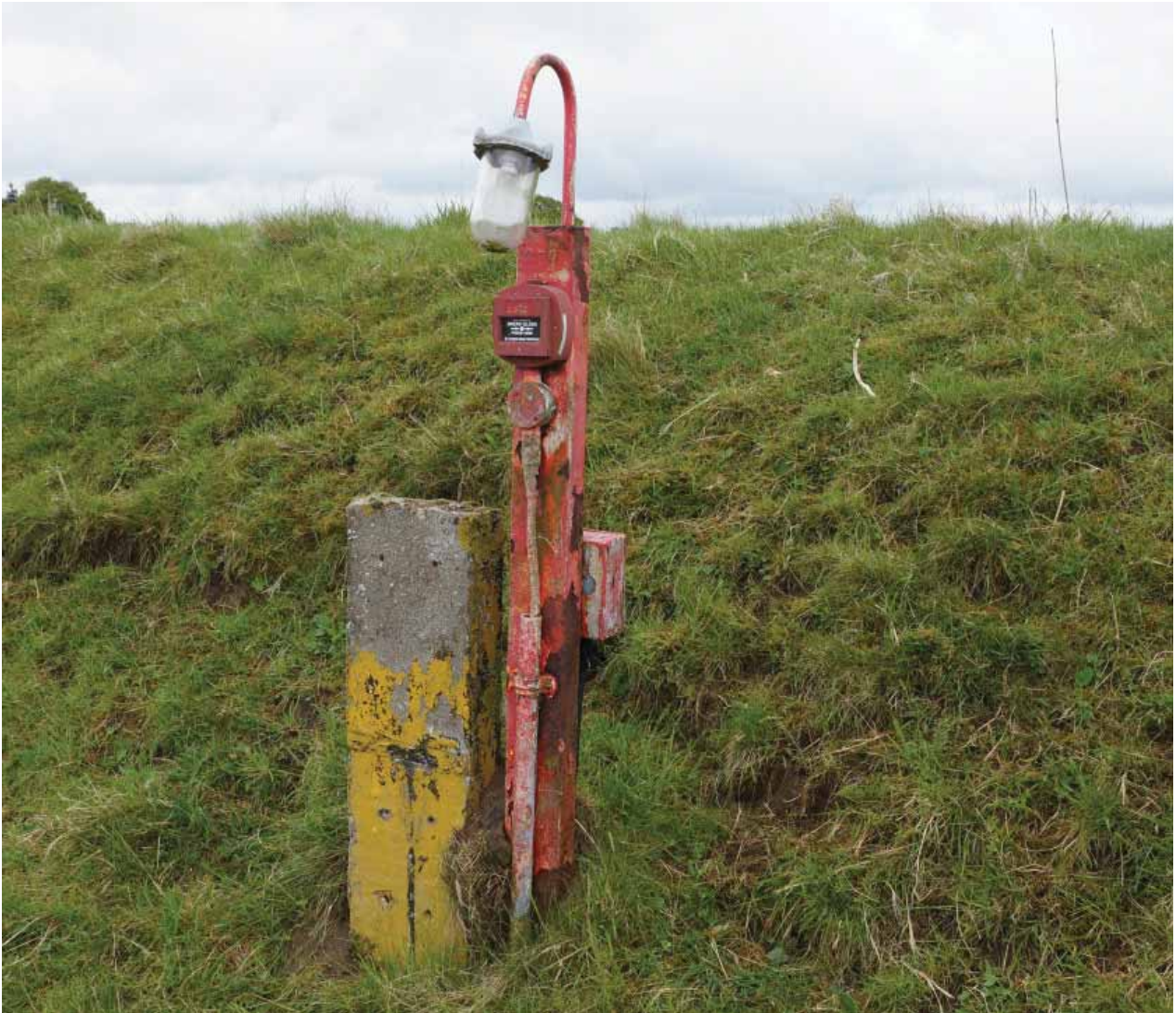
Plate 46: Fire alarm station
