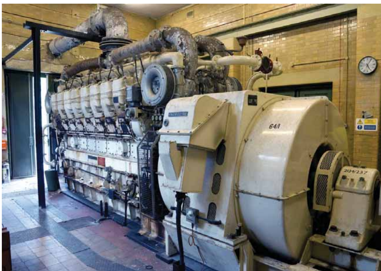
Plate 38: Standby set house (58), English Electric diesel engine
