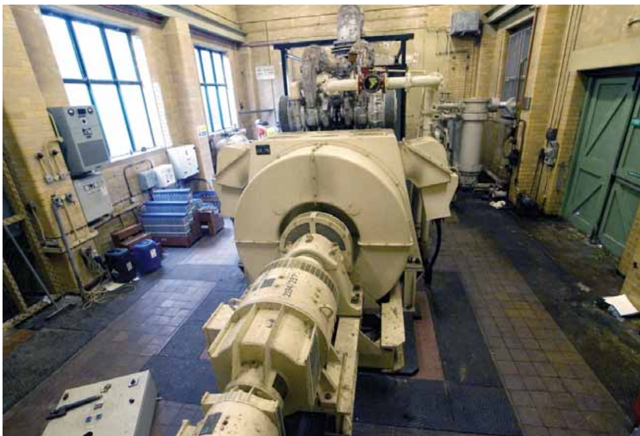
Plate 37: Standby set house (58), English Electric diesel engine
