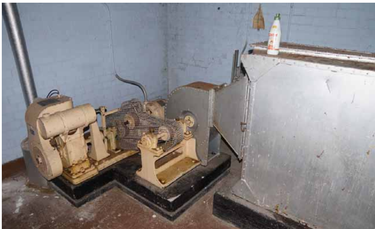
Plate 14: Station sick quarters annexe (33), view showing original plant This is a Lister engine-driven blower and filter pack
