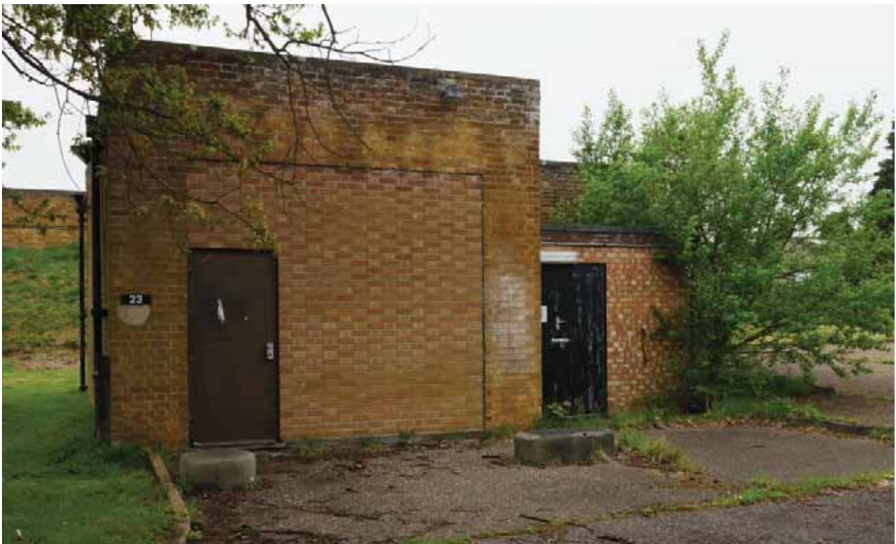
Plate 1: Ambulance shed and mortuary (23), front elevation Showing the main entrance to both the garage and mortuary bricked up and smaller doors inserted.
