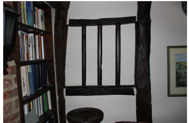
Old mullion window incorporated into newer wall.
