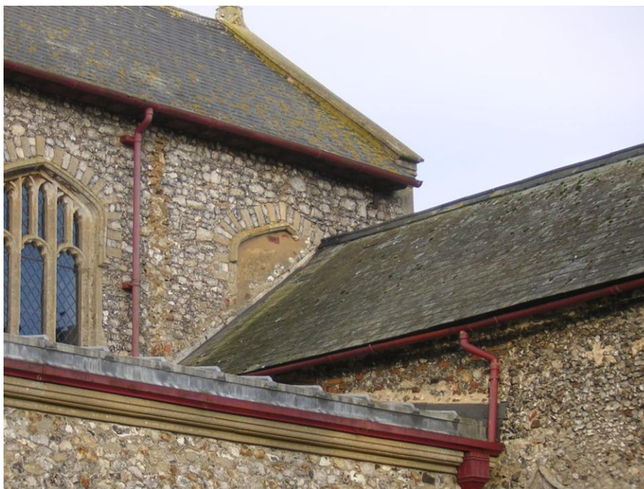
Church showing original window which has been blocked and then partially covered by an extension.
