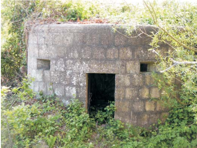
First World War pillbox at Wayford Bridge, Stalham
