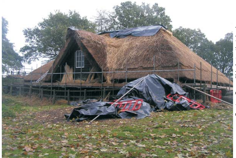
Gunton Sawmill being rethatched
